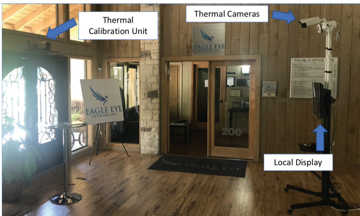
▲ Figure 5: Thermal camera setup in an office lobby
